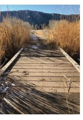
John Campbell took on two other fall maintenance projects. He patched the holes in the one footbridge damaged some time ago by a horse. John considered this a temporary solution to fix the safety issue and advised that replacement floor boards will need to be laid in the spring. John also inspected the high ditch, looking for any debris that needed to be removed.
